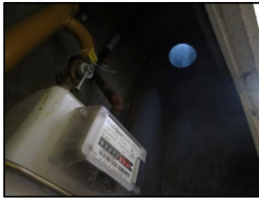
Photo N° 344 AMIANTE CIMENT -- GAINTE TECHNIQUE 4 Gainses & coffres horizontaux Ventilation haute (Fibres-ciment)
