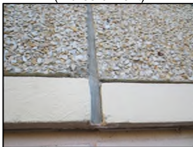
Photo N° 360 ECH-N°2 FACADE Murs Joint dilatation
