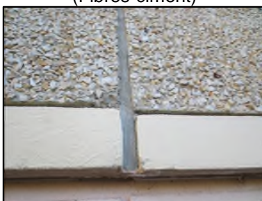
Photo N° 360 ECH-N°2 FACADE Murs Joint dilatation
