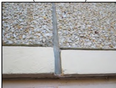
Photo N° 360 ECH-N°2 FACADE Murs Joint dilatation
