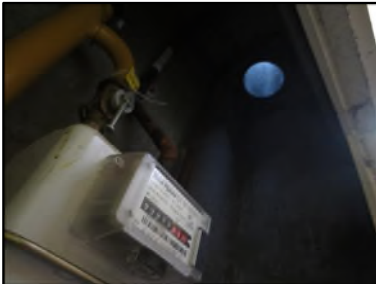
Photo N° 344 AMIANTE CIMENT -- Gaine technique 8 Gainses & coffres verticaux Ventilation haute (Fibres- ciment)
