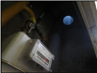
Photo N° 344 AMIANTE CIMENT -- Gain technique 8 Gains & coffres verticaux Ventilation haute (Fibres- ciment)
